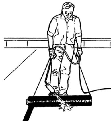
Fig. 2 Welding of Derbigum GC to primed concrete substrate
